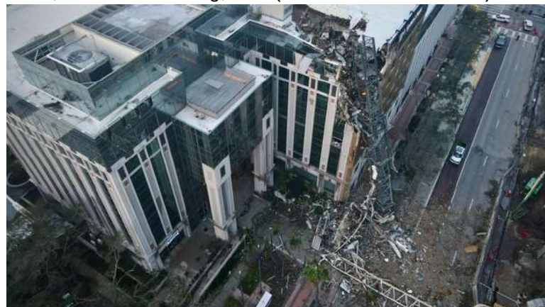
The roof of the Tropicana Field is damaged the morning after Hurricane Milton hit the region, Thursday, Oct. 10, 2024, in St. Petersburg, Fla. (AP Photo/Julio Cortez)
